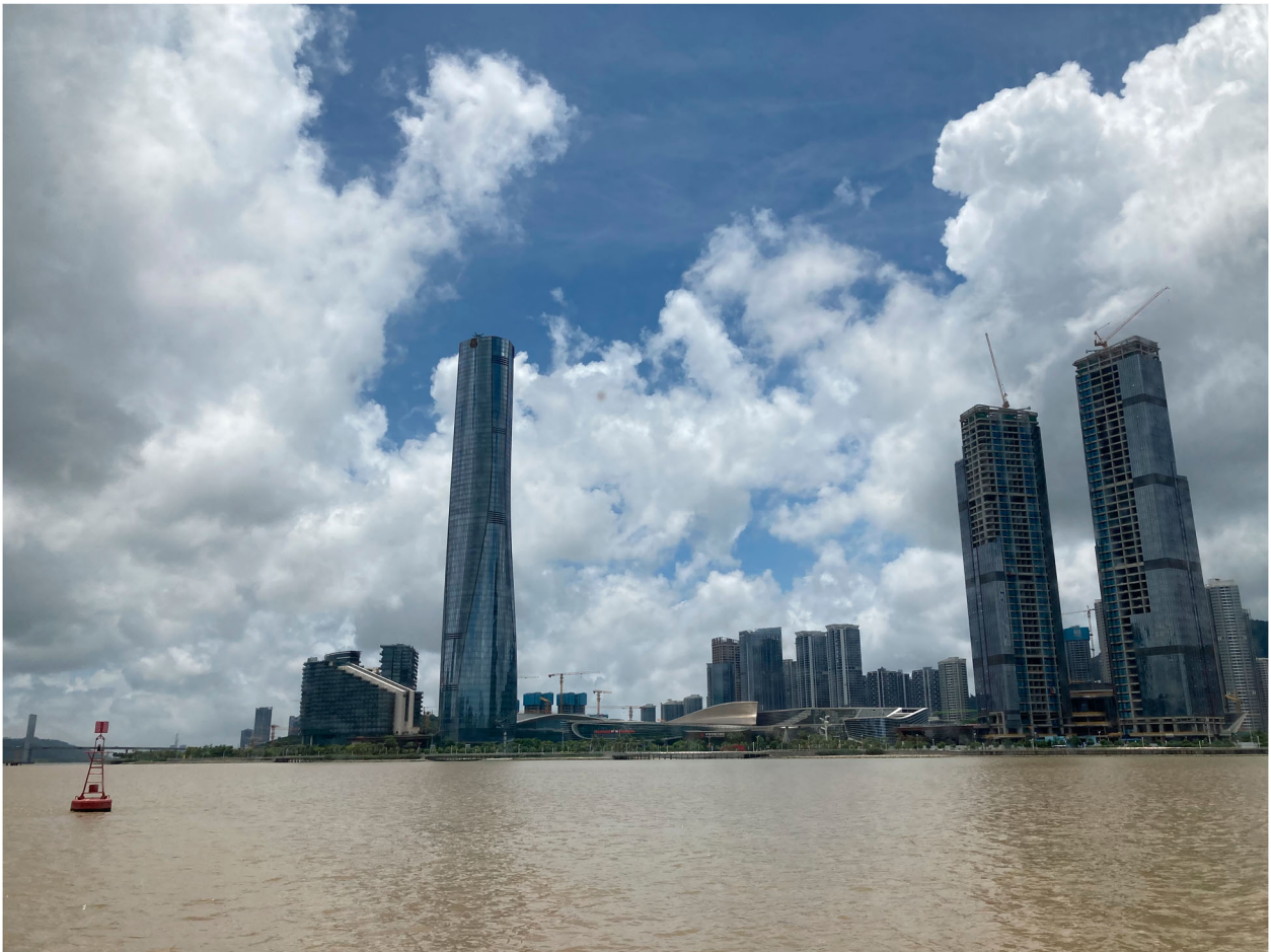
FIGURE 6. Hengqin Central Business District under construction. Photo: Authors.
